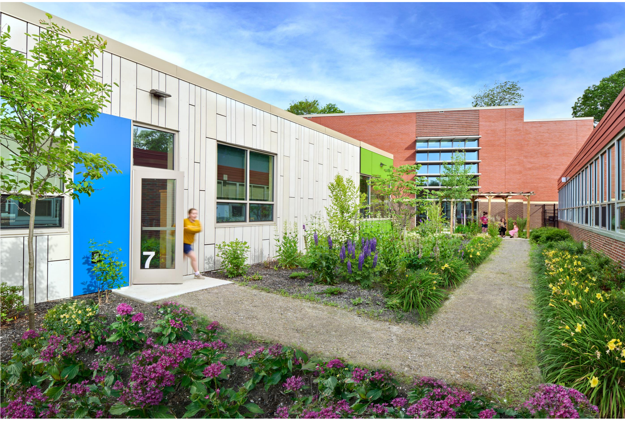
Diverse secure interior courtyards allow for group and individual connections to nature. The library courtyard provides a respite for reflection, play and learning.
